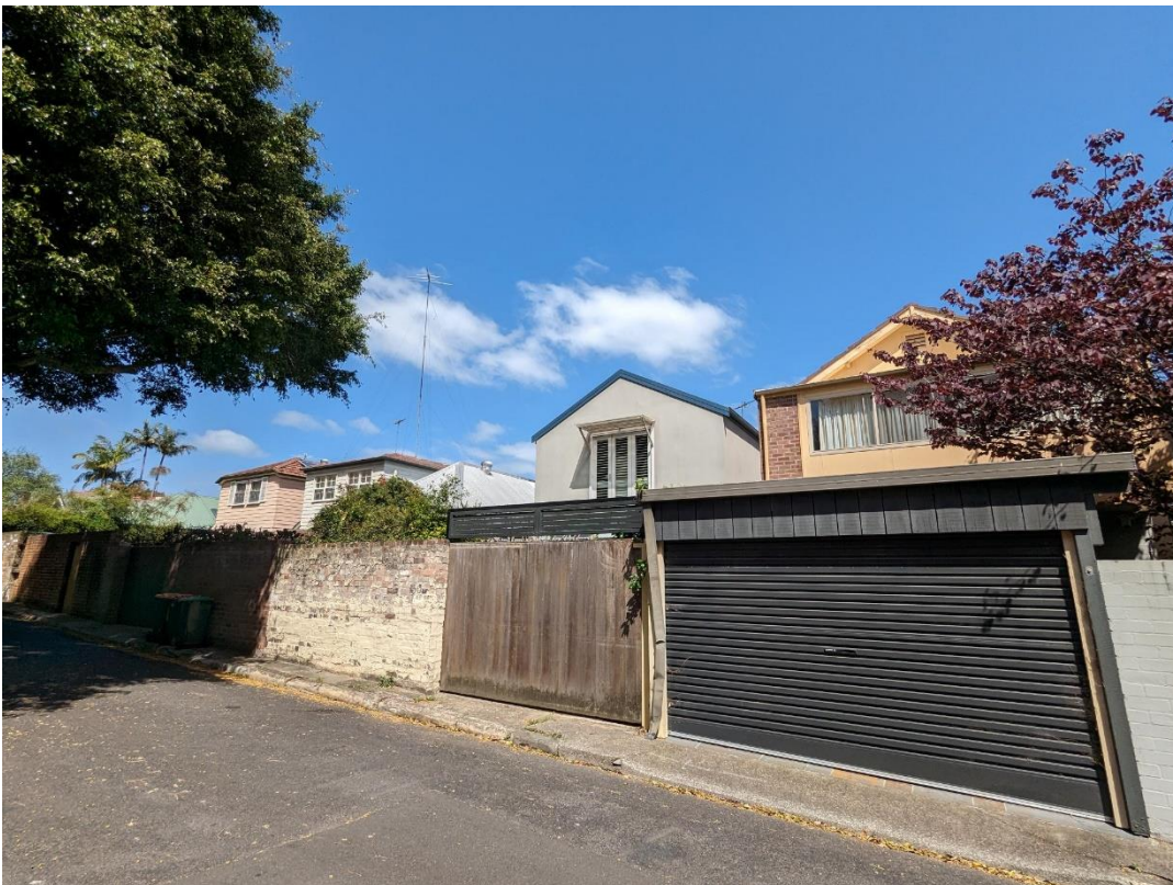
Figure 12: Neighbouring developments with two storey rear additions on Allen Lane
